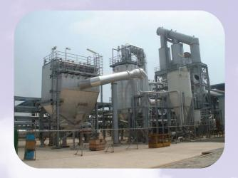
"Dry" Scrubber using bagfilter and hydrated lime Ca(OH<sub>2</sub>) injection to remove fine particulate and neutralize acid gases. No wastewater treatment requirement
