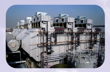
IWS<sup>TM</sup> ionizing wet scrubber for the simultaneous removal of fine sub-micron sized particulate and gas phase pollutants.
