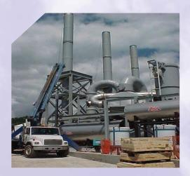
3\*100 MBTU/hr fume and liquid waste incinerators with waste heat recovery and gas cleaning
