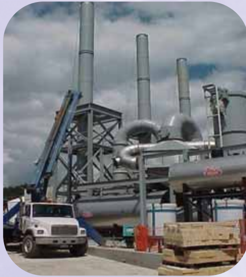
Three 100 MBTU/hr fume and liquid waste incinerators with waste heat recovery and gas cleaning for pharmaceutical plant in Puerto Rico.
