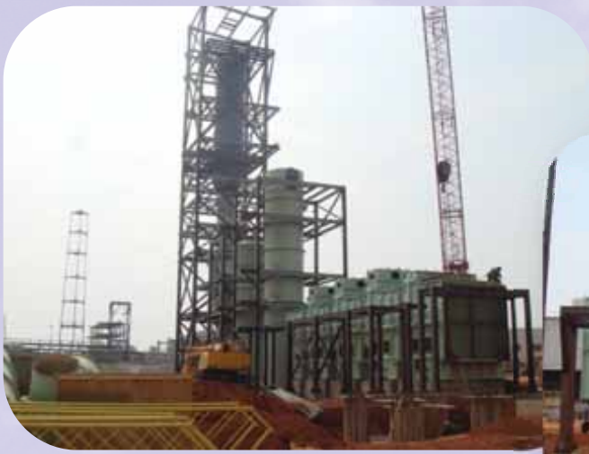
60 GJ/hr vertical Incinerator with Gas Cleaning for treatment of gaseous and liquid Chlorinated Silane Wastes for Silicone/ Siloxane plant in China.
