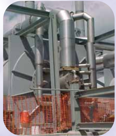
Three 100 MBTU/hr fume and liquid waste incinerators with waste heat recovery and gas cleaning for pharmaceutical plant in Puerto Rico.
