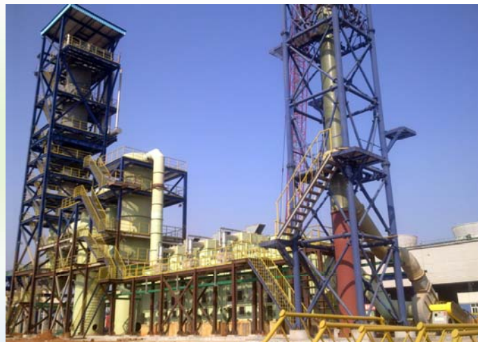
From Left to right: Incinerator, Quench, Ventruri, Condenser, IWS™ Scrubber, Fan and Stack.
